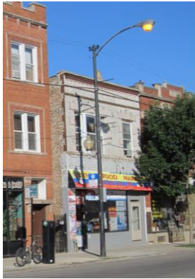
Existing Former Conventional Roadway Light Pole
